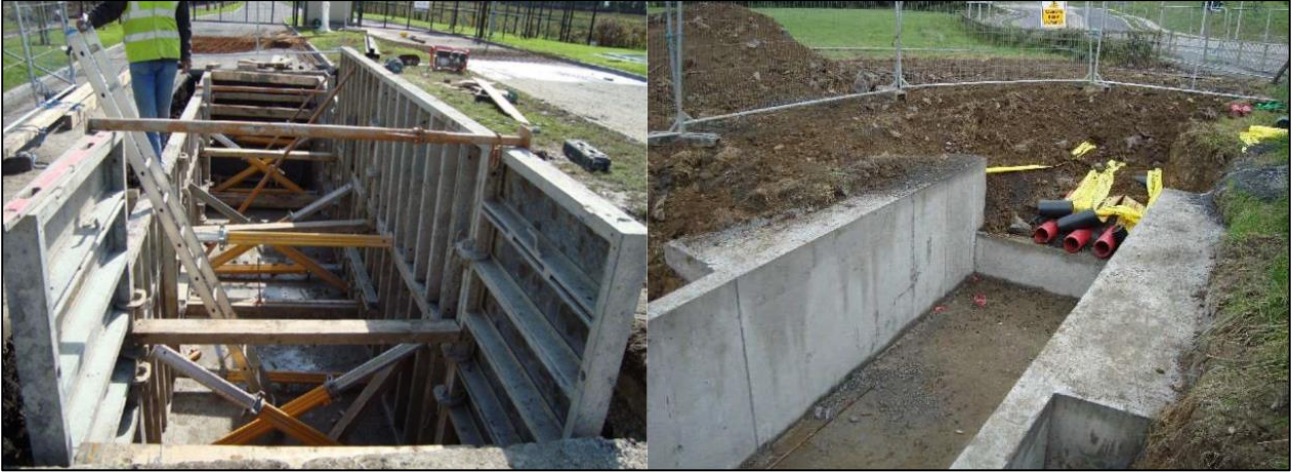
Figure 2-4: Typical Joint bay installation.
